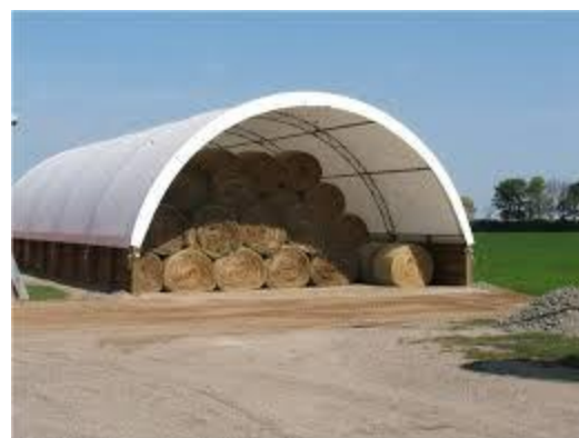
Fabric Structure Hay Shed Photo: Four Winds Builders, LLC
